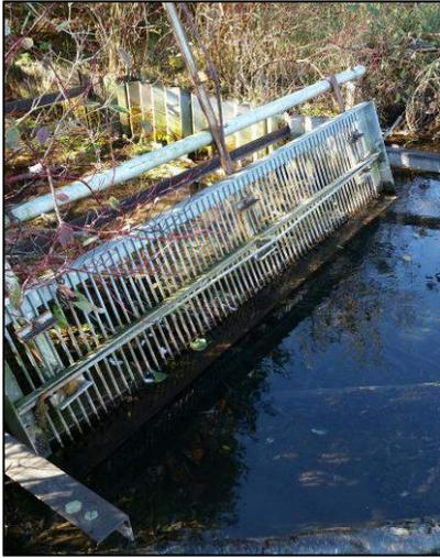
Image 3. Partial Fish Barrier, upstream reach of segment 3.
