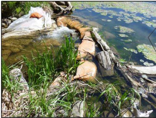
Image 5. Partial Fish Barrier, north upstream reach of segment 7.
